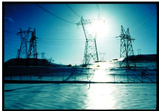
Figure 13: High Voltage Transmission Towers
