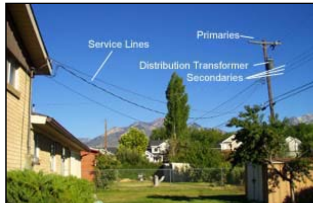
Figure 23: Household Service Line Drop from Distribution Line
