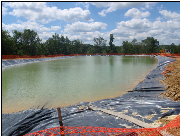
Lined Fresh Water Supply Pit from the Marcellus Shale Development in Pennsylvania
