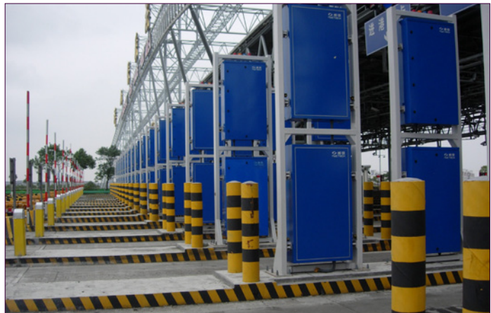
The 17 radiation portal monitors installed at the Port of Yangshan will scan 100% of export containers.
