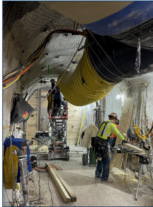
The crafts needed to complete the horizontal concrete plug included carpenters and ironworkers who built the bulkheads needed to support five separate grout pours over five months.
