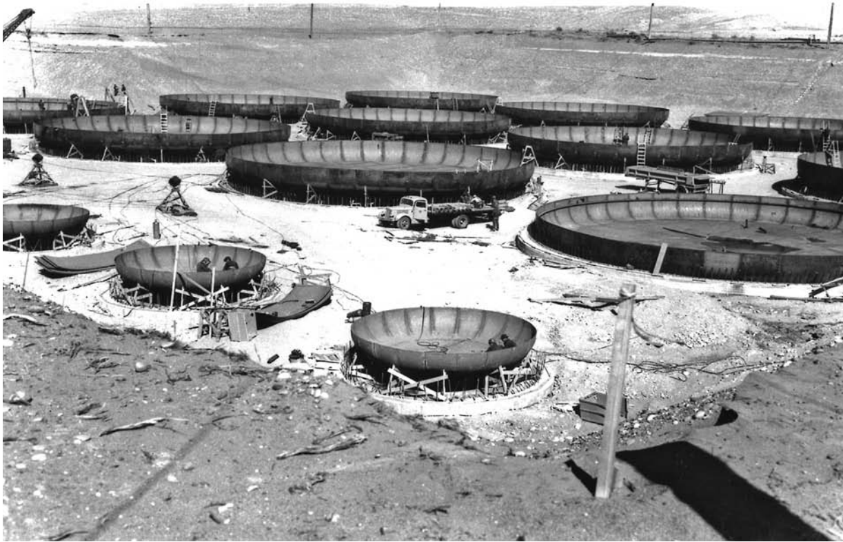
241-T tank farm under construction, early 1944
